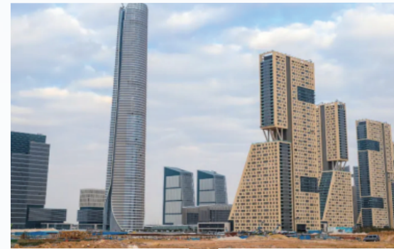
Egypt's New Capital CBD Project
